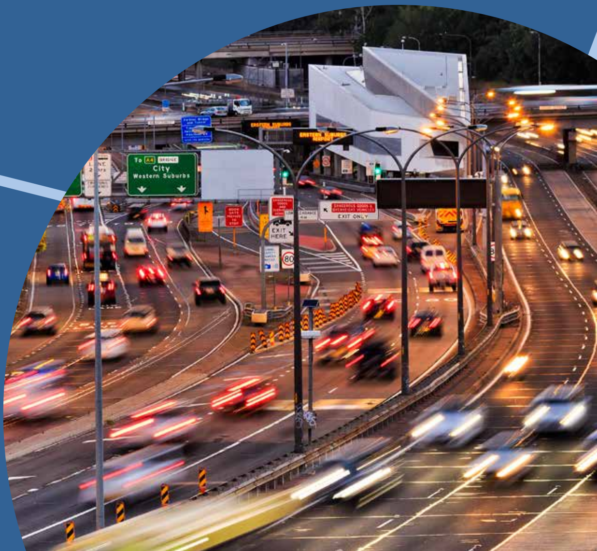
Warringah Freeway Sydney, NSW
